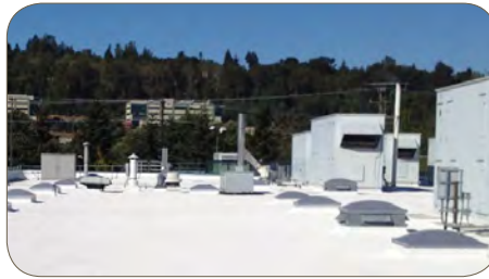
Title 24 reflective roof and prismatic light-gathering skylights at the South Base Maintenance building.
