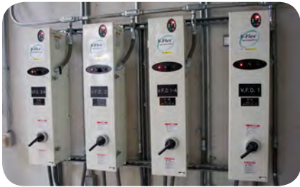
Variable frequency drive fan controls for Ryerson Base save energy by running motors at less than 100% output when full power isn't needed.
