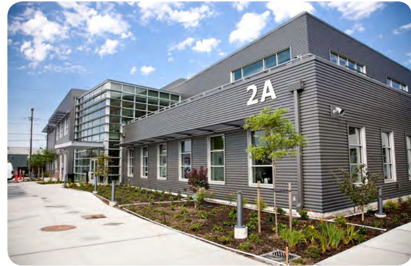
The LEED Gold certified Atlantic/Central Operations Base includes highly reflective roofing and paving, an exterior vegetated wall that provides shading for the west façade, native vegetation, low-flow water fixtures and natural daylighting.
