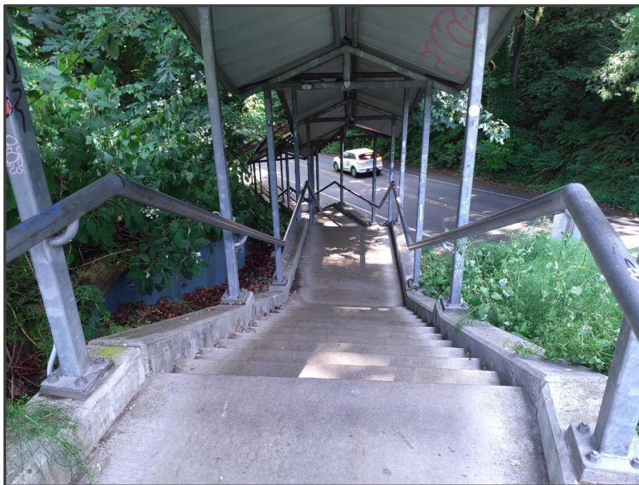
Figure 12: Staircase at Vashon North End Park-And-Ride
