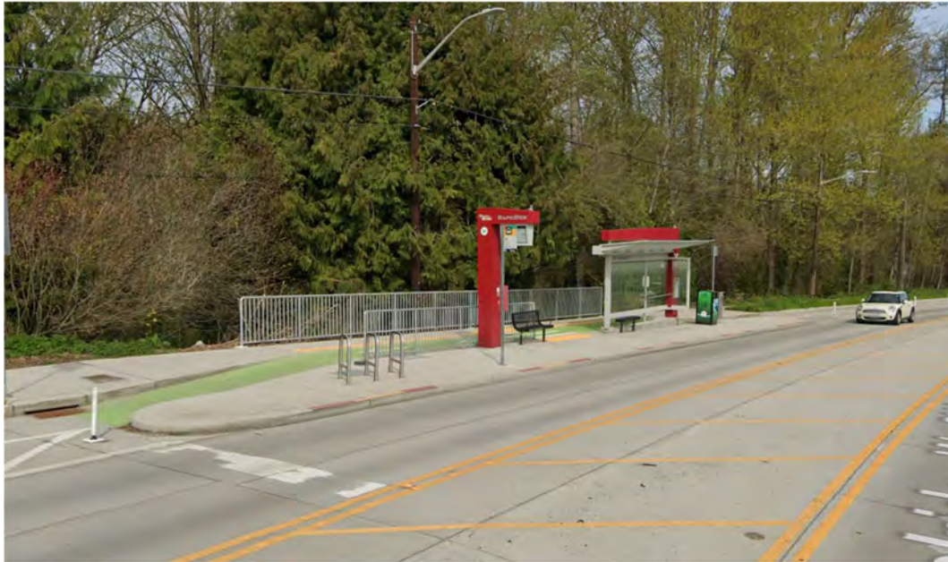
Figure 20 Example Transit Boarding Islands on the RapidRide H Line
