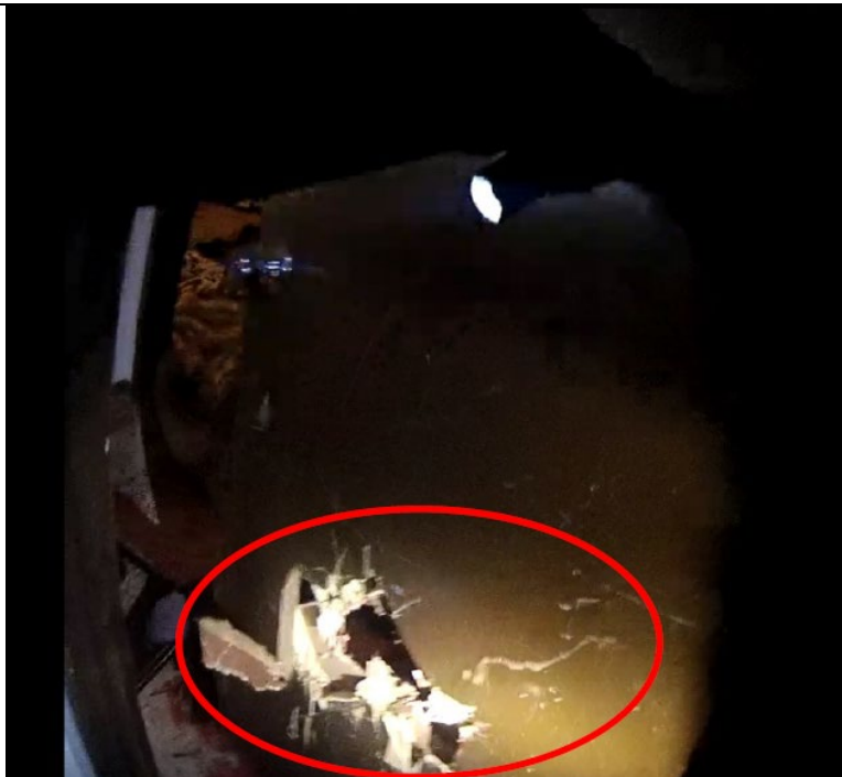
Figure 3 - Screenshot of Involved Officer 1's BWV, which shows the damaged door prior to officers forcing it open. Inside the room, officers located Rodriguez Martinez and Victim 1.
