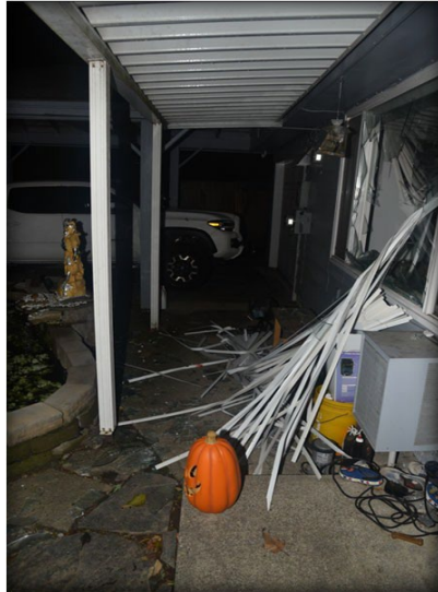
Figure: Photo is of the shattered picture frame window.
