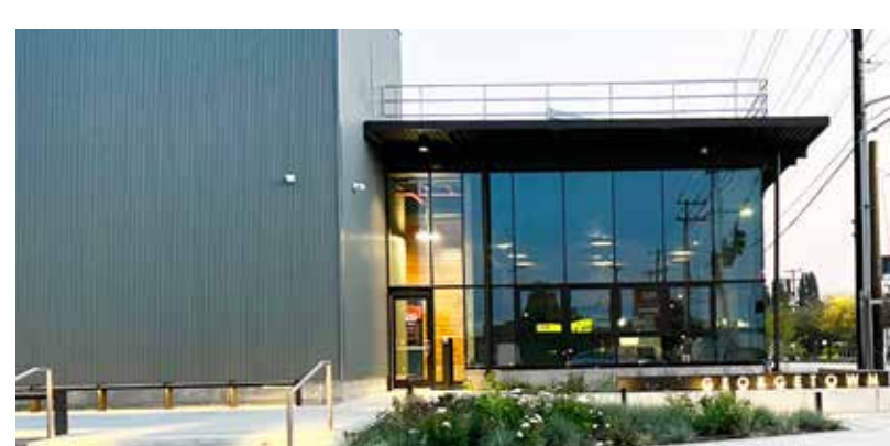
The Georgetown Wet Weather Treatment Station is a newly completed CSO control facility that will treat up to 70M gallons per day of sewage and stormwater during heavy rains to protect the Duwamish River. It will control two King County CSO outfalls: Brandon and South Michigan. Construction was completed and the facility was put into operation in 2022.
