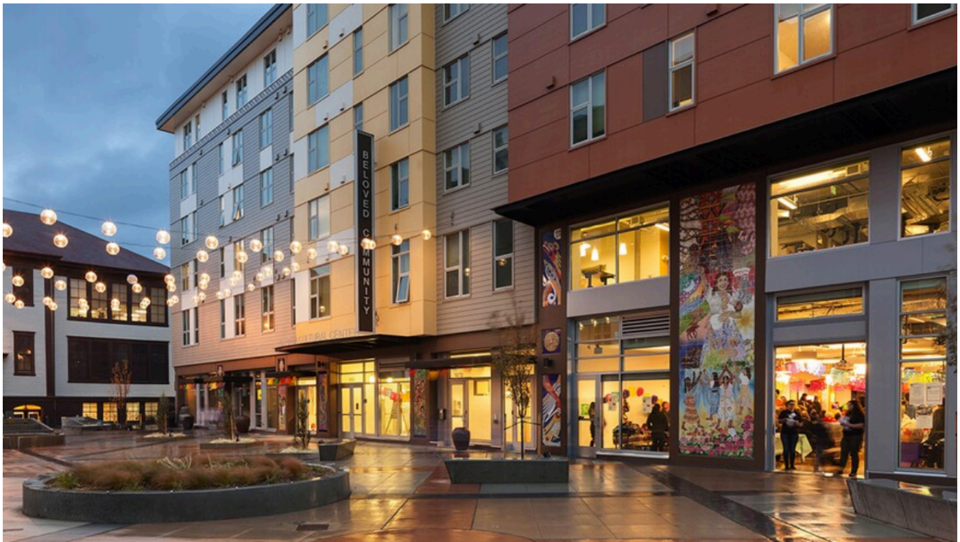
Roberto Maestas Plaza has a strong architectural concept that connects a central plaza with adjacent active uses and culturally rich art related to the Centro de la Raza. 7 Directions Architects/SMR
