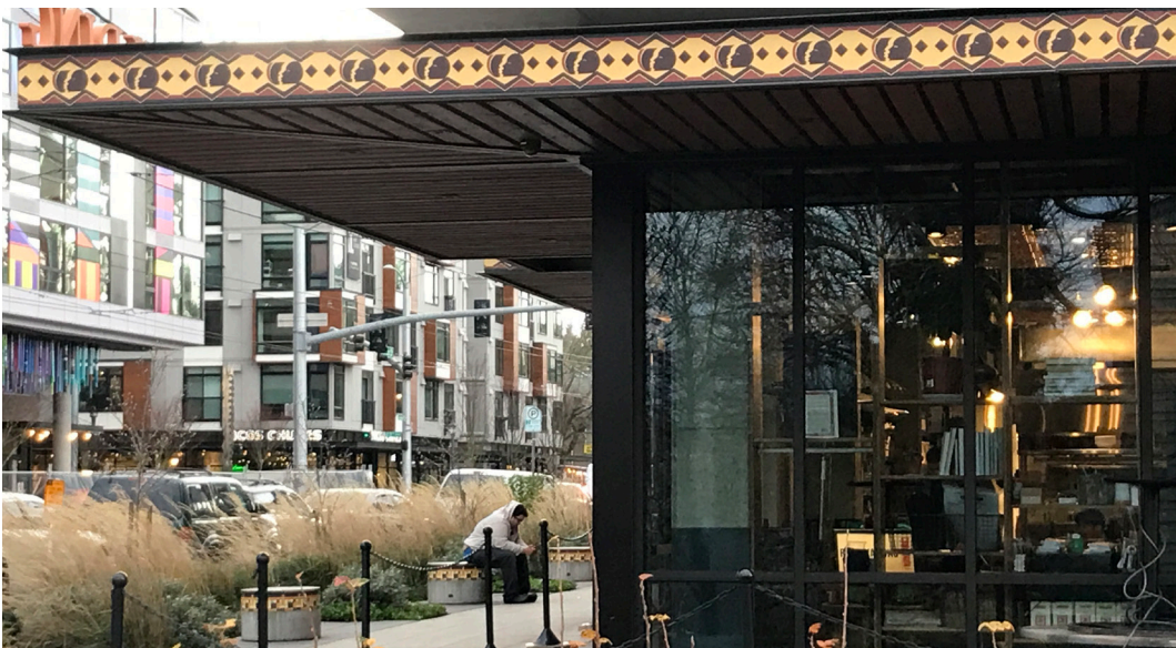
This building at Seattle's Central District include details on the canopy edge incorporate by African art motifs.
