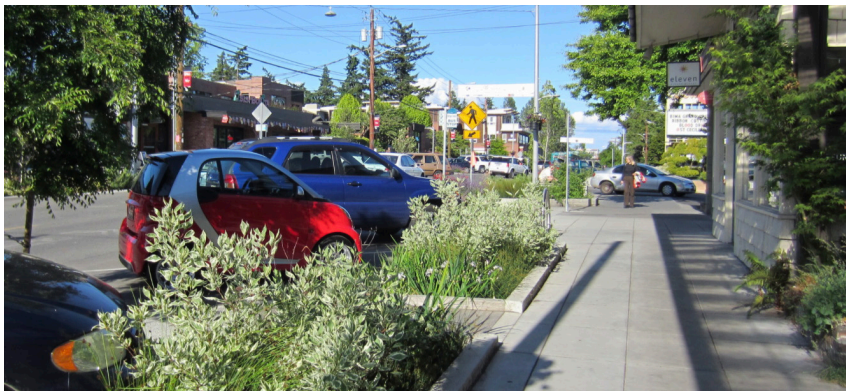
Examples of beautiful stormwater treatment in an urban setting. (SvR/MIG)
