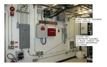
VIEW NORTH INSIDE BUILDING SHOWING CABLE ENTRY PANEL, INTERIOR GROUND BAR, AND CONDUIT EGRESS POINT
