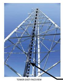
7/8" COAXIAL CABLE PATH -USE SITEPRO1 SR78-K CUSHION HANGERS AND ADAP-O ANGLE ADAPTERS WITH 36" MAXIMUM SPACING FOR HORIZONTAL RUN AT TOP
