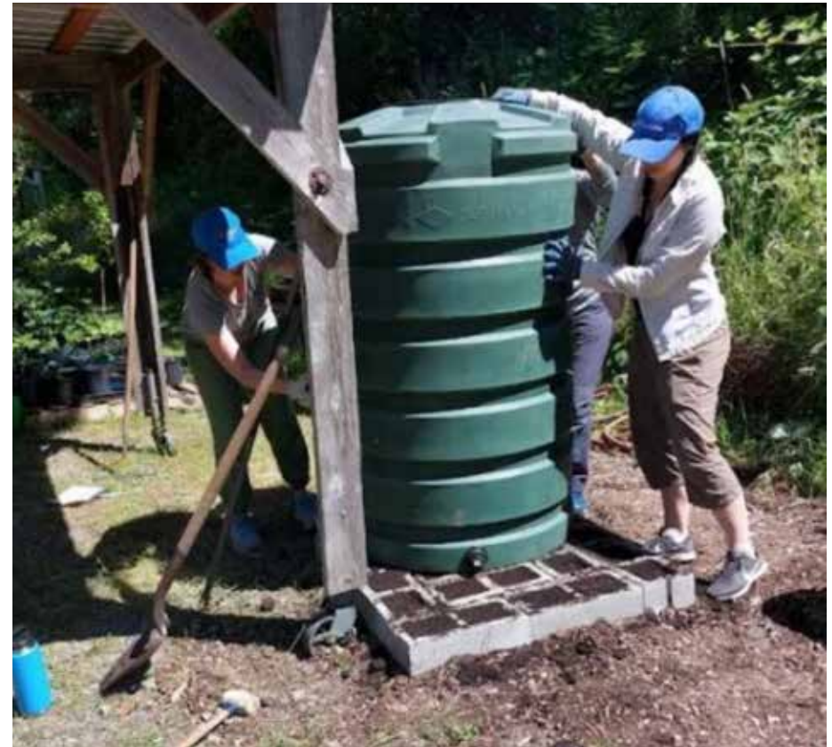
Participants in the Soil and Water Stewardship training install a cistern at the Rainier Beach Urban Farm.
