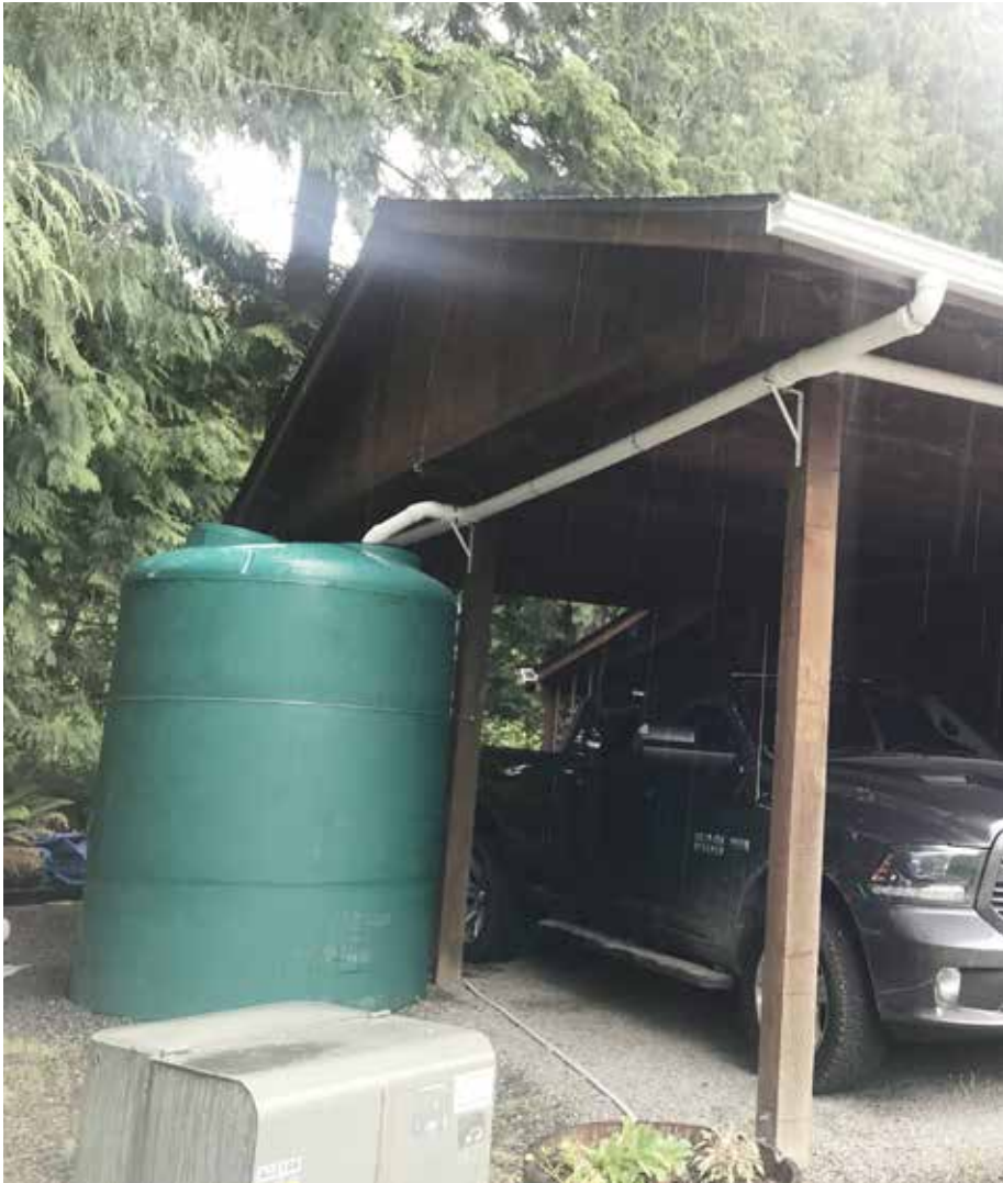
Cistern number one installed on the side of the garage/shop.
