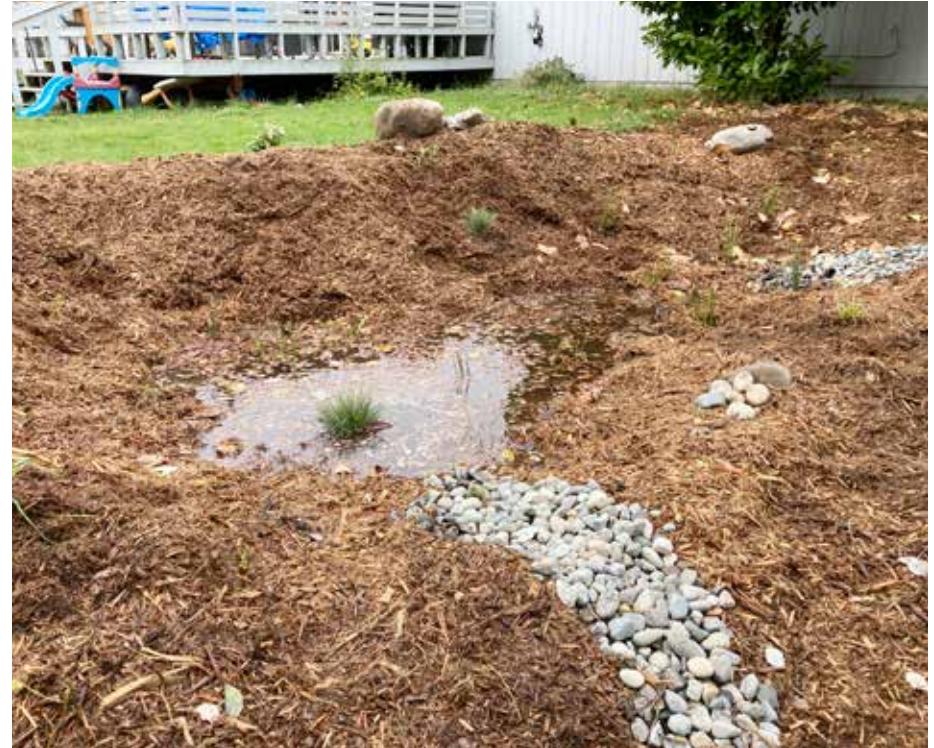
Rain garden installed on White Center property.
