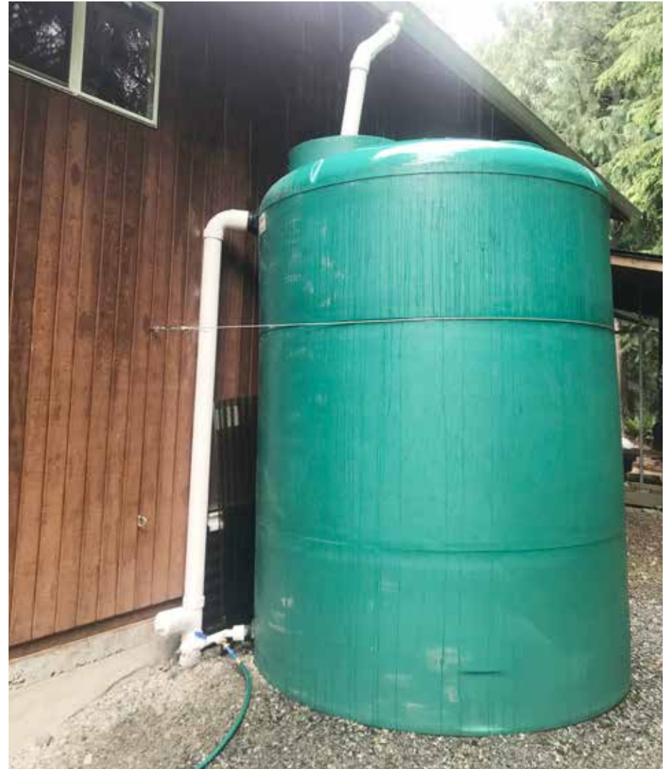
Cistern number two installed behind the garage/shop.
