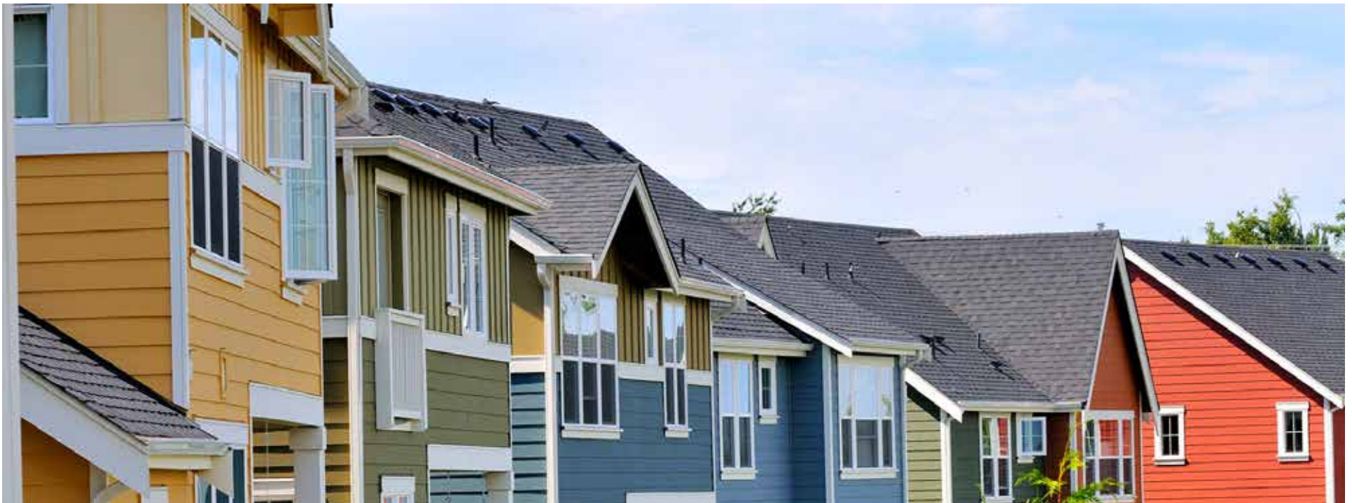
Seattle Housing Authority RainWise Big Roof program at High Point.
