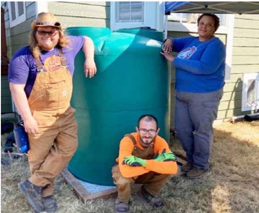
Green Start Crew installing a residential cistern.
