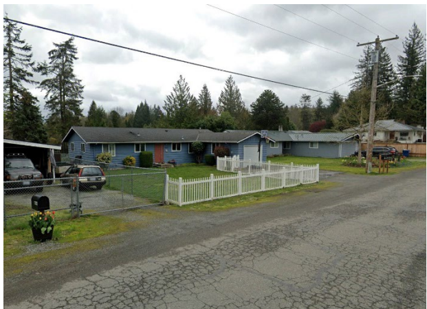
Figure 21. One-Story Ranch Home with Attached Garage
