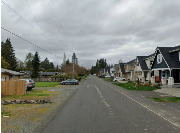
Figure 32. Wide Paved Street without Curbs
