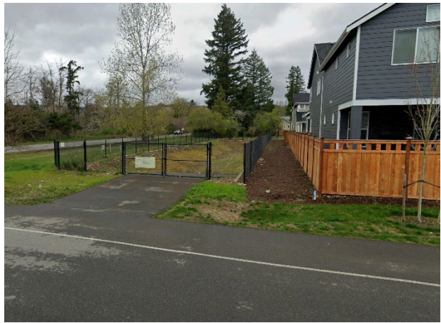
Figure 33. On-site Stormwater Pond
