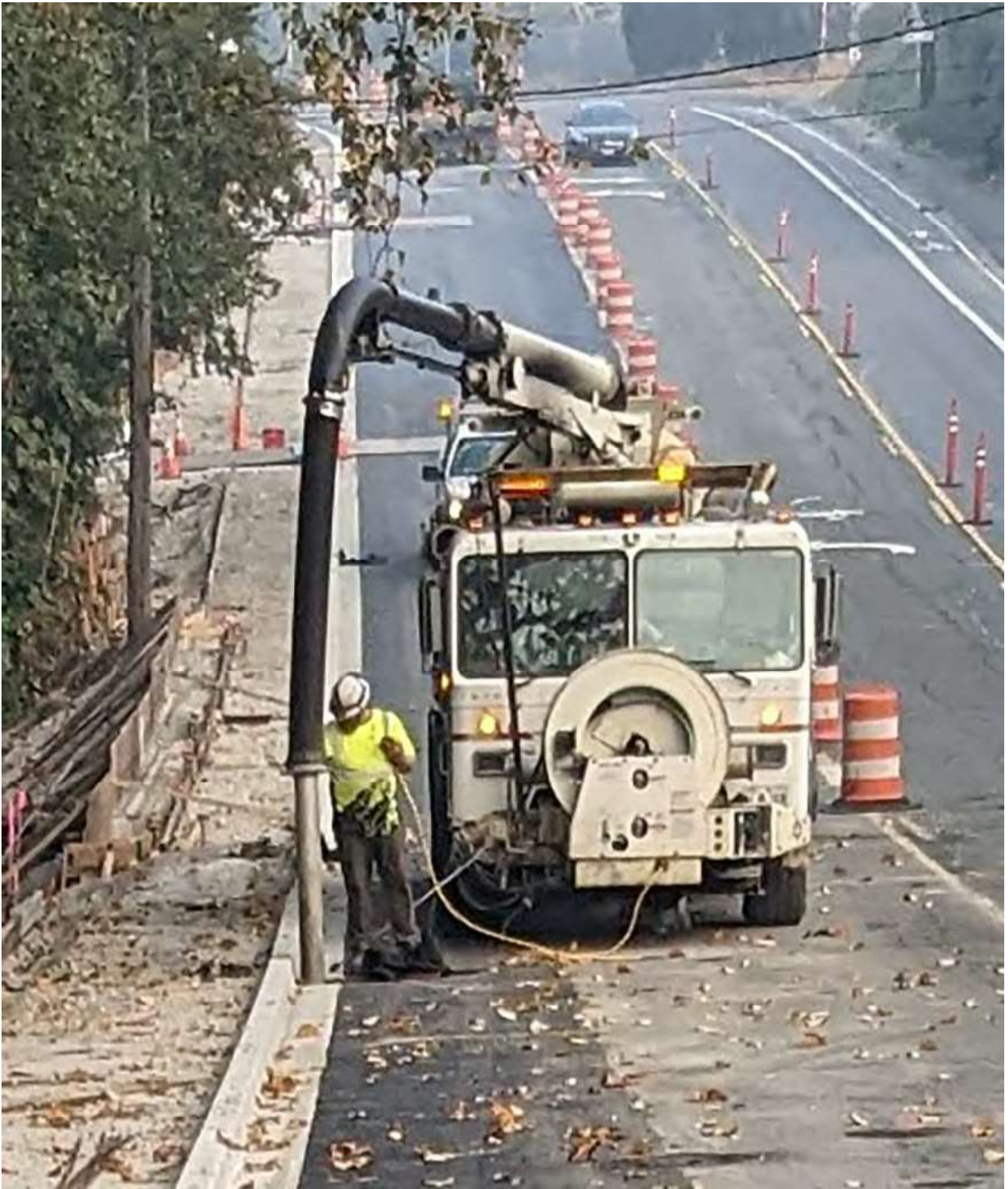
Oct. 19, 2022 – It takes a massive hose to suck up any construction debris to clean the freshly poured gutter and curb. This makes sure the new drainage system is ready for wet weather.
