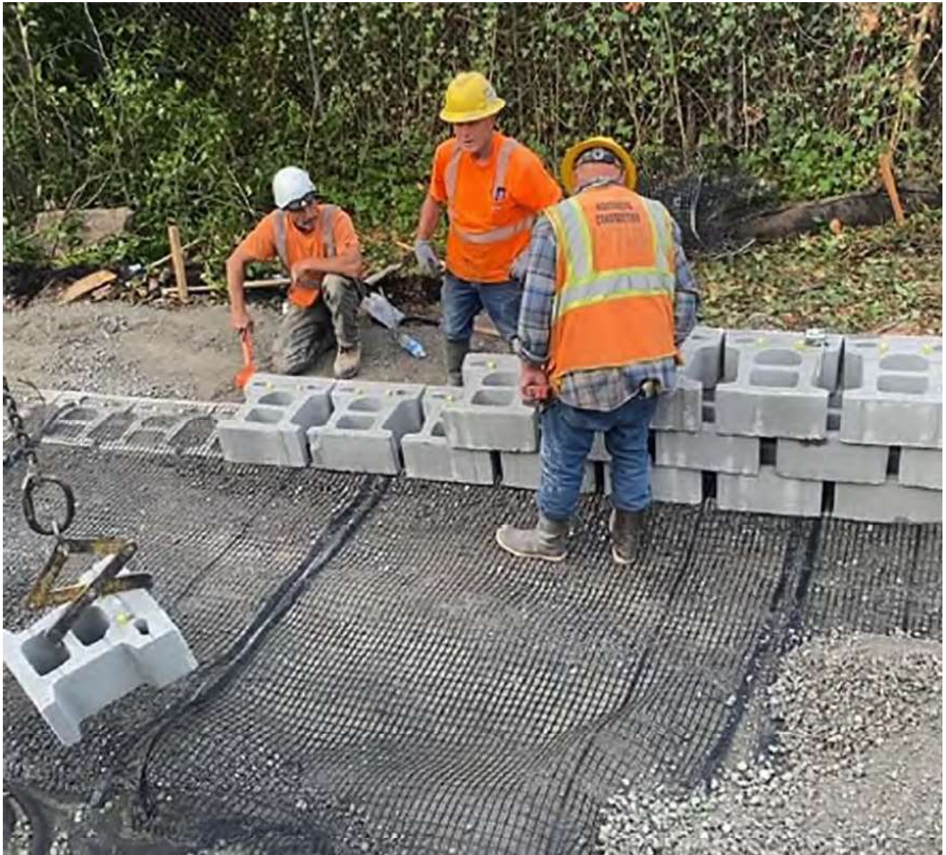
Oct. 5, 2022 – Crew members build a supportive wall for the sidewalk which will go down Renton Avenue S.
