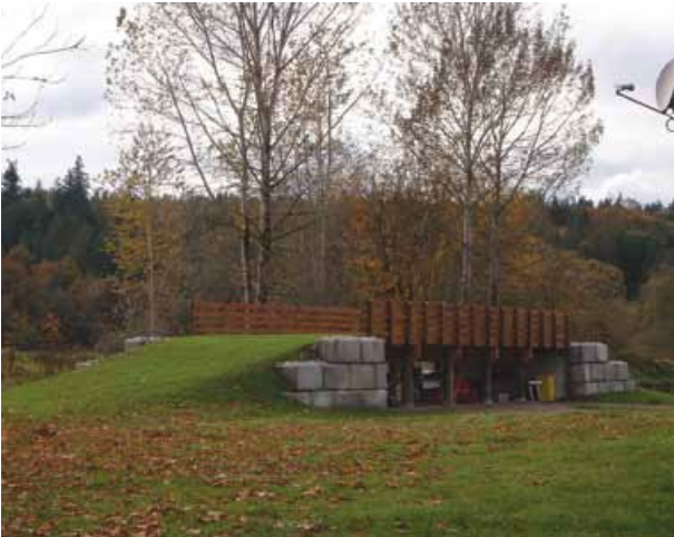
Figure 22. Barn Elevation Pilot Project Platform
