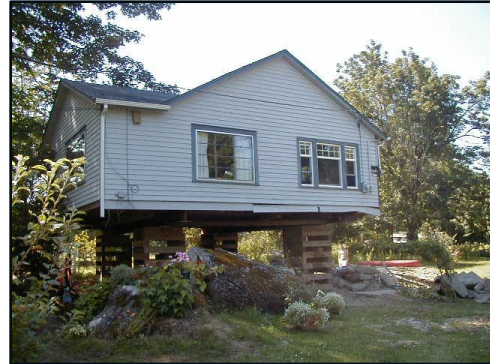
Figure 21. Home Elevation Project During Construction
