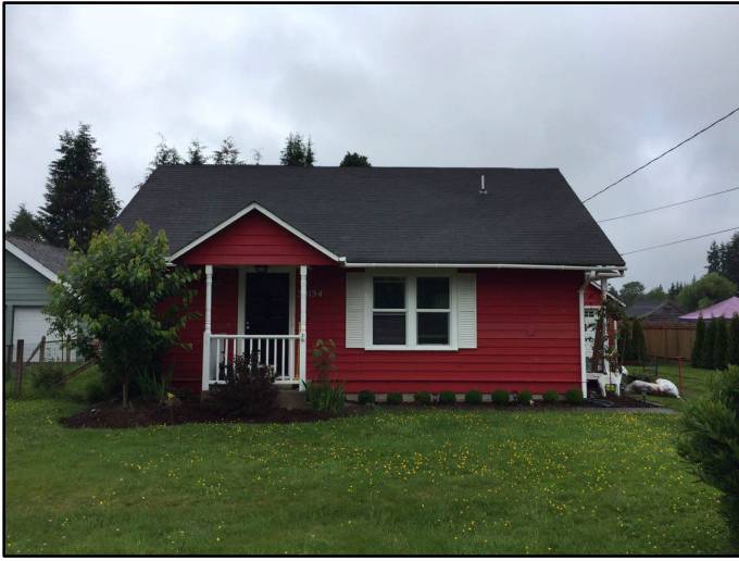
Figure 18. Before Home Elevation, 2015
