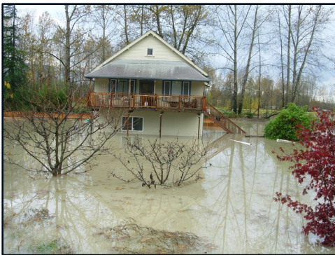
Figure 20. Elevated Home with Flooding, Nov. 2006
