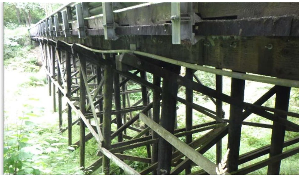
Figure 27. Ames Lake Trestle Bridge No. 1320A
