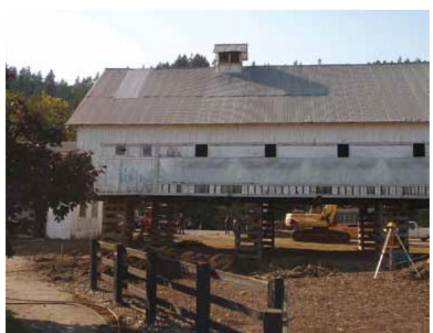
Figure 23. Barn Elevation Pilot Project Livestock Barn
